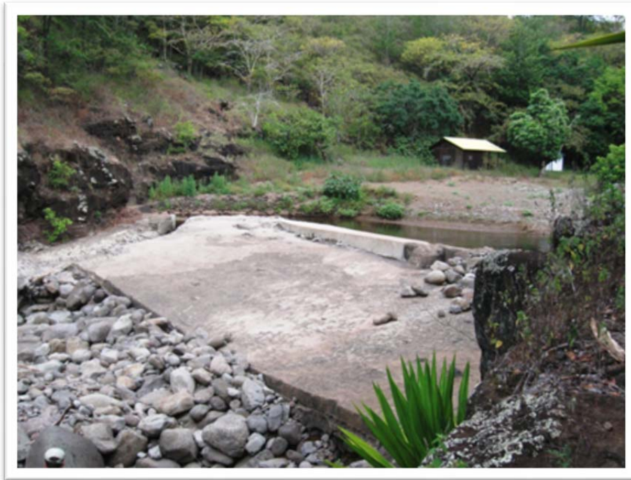
Waiahulu Dam, view from east
