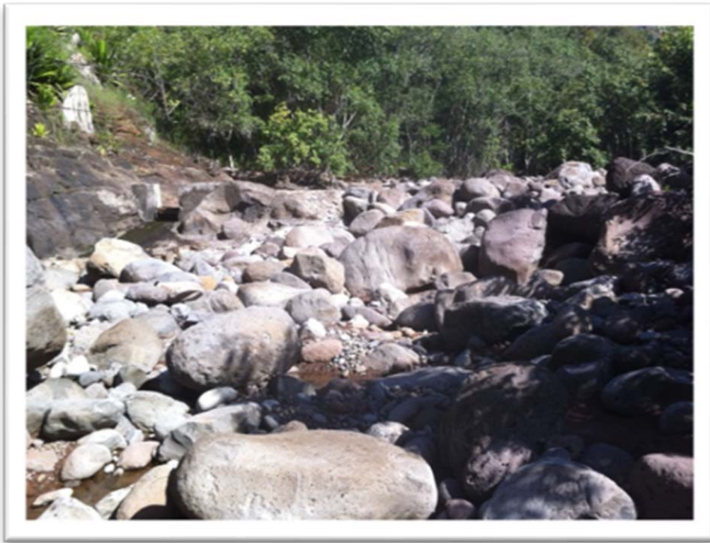
Below Koai'e Dam (outlet at left)
