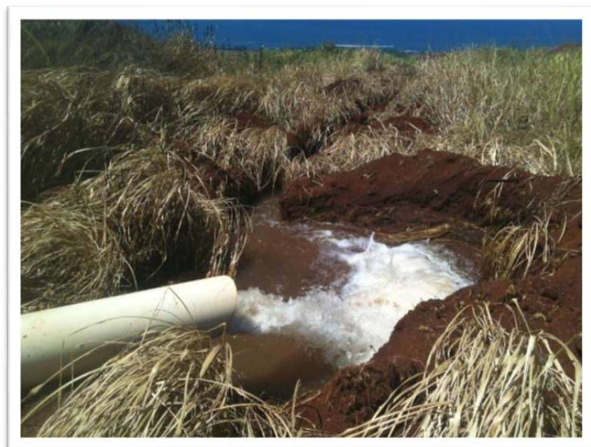
Redirected dumping from Kōke'e Ditch
