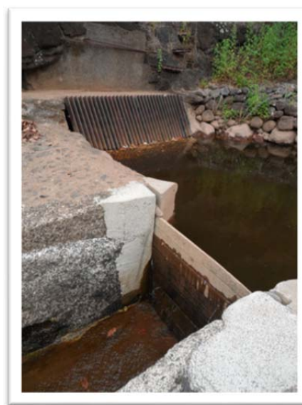
Waiahulu Dam diversion grate and boarded-up outlet
