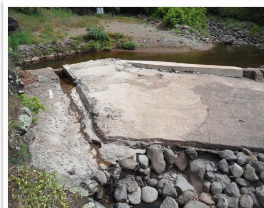
Waiahulu Dam (boarded-up outlet in middle left)
