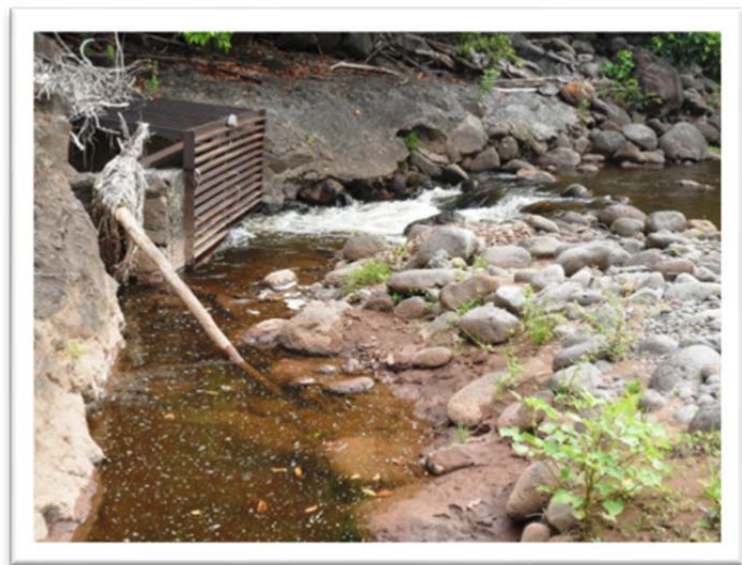
Koai'e diversion, looking from top of dam
