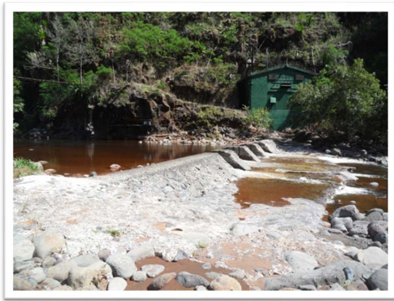
Mauka Powerhouse Dam
